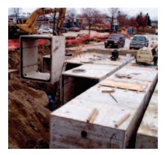
keyed ends, sloped-faced ends and watertight joints. Optional exterior coatings can also be applied at the plant, reducing on-site construction. Precast concrete box culverts can be produced in any size limited only by transportation weight.
